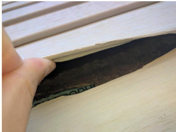
Vinyl Deteriorating
