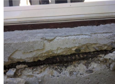
Exposed Rebar
