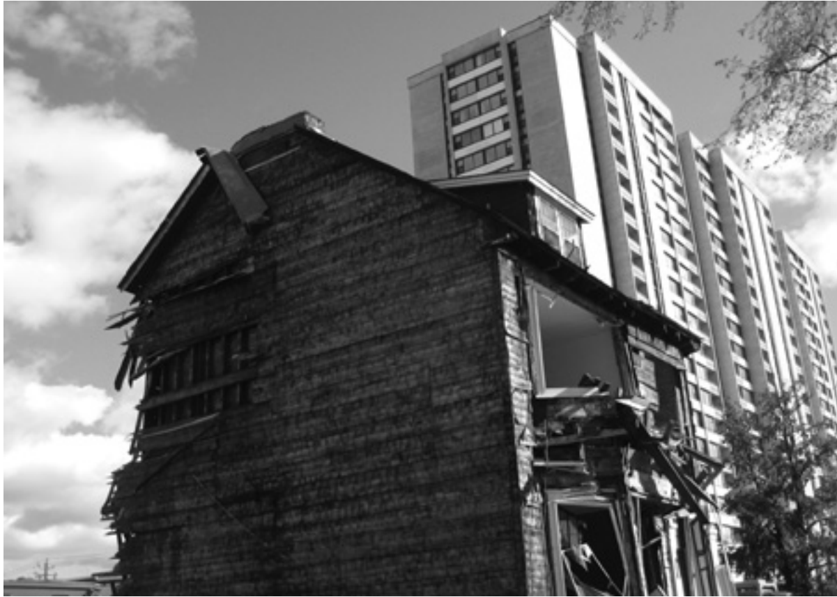
Heritage South Park home demolition for Trillium Project (photo Kim Thompson)
