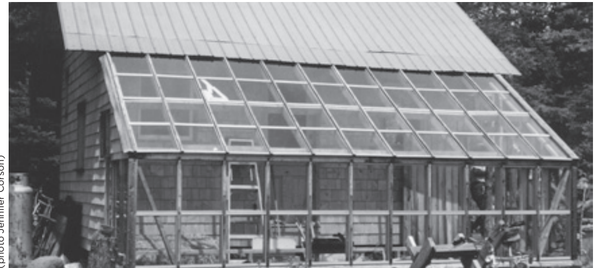
Greenhouse constructed using old windows (photo Jennifer Corson)
